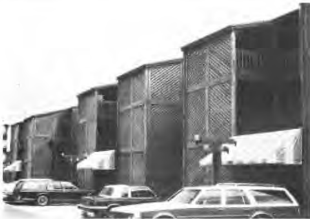
Figure 3.32. The diagonal battens used to enclose the stairwells for protection provide an aesthetically appealing screen-textural affect. The colored awnings also add a necessary highlight to an otherwise colorless exterior. Notice also the pole light fixture.
