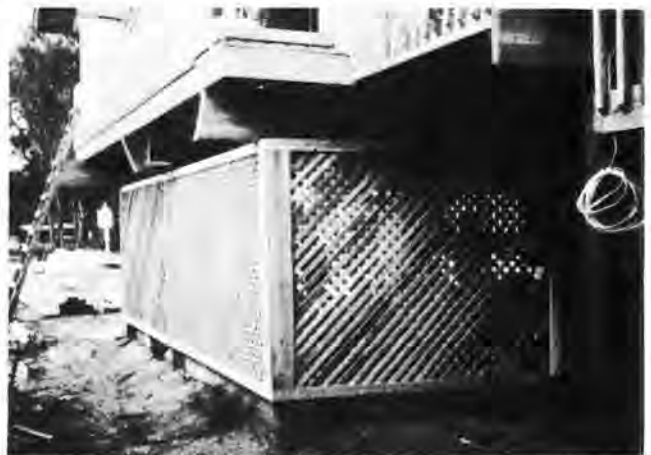
Figure 4.54. Breakaway Walls
