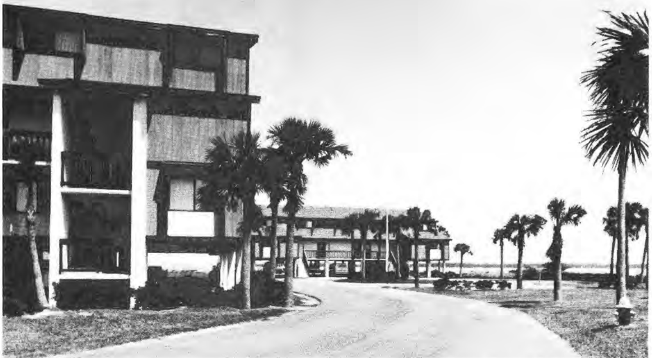
Figure 3.34. This structure uses a mixture of materials, texture and color very successfully and provides a variety of form for visual appeal. The space under the building remains open and light through a combination of white unobstructed walls and piers, landscaping, and layout relative to other buildings. A human scale is accomplished by breaking the building up into different heights and sections, rather than an imposing three-story box, as is often done (see also Figures 3.58 through 3.62).
