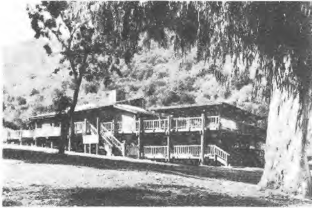
Figure 3.25. This wood structure successfully uses the same material throughout the building—foundation, structure, treatment of railings, wall, and roof material, as well as connection and anchorage details. The design honestly expresses the structure, foundations and other building elements. While it is obvious this is an elevated structure, it still feels very much a part of the site. The foundation members are also integrated well with the building itself (see also Figures 3.54 to 3.57).
